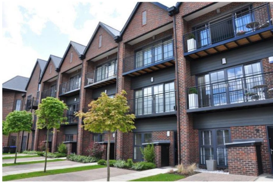
(8) Balconies and terraces provide suitable levels of private amenity space within flatted developments
